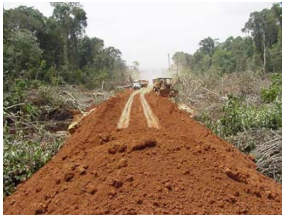
Figure 21: Illustration of road construction works across a swamp
