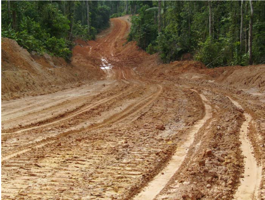
Figure 2: Photograph of a road segment showing clayey soils
